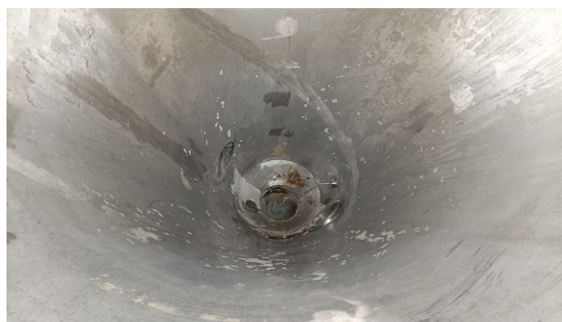
Slurry service tank (after)
