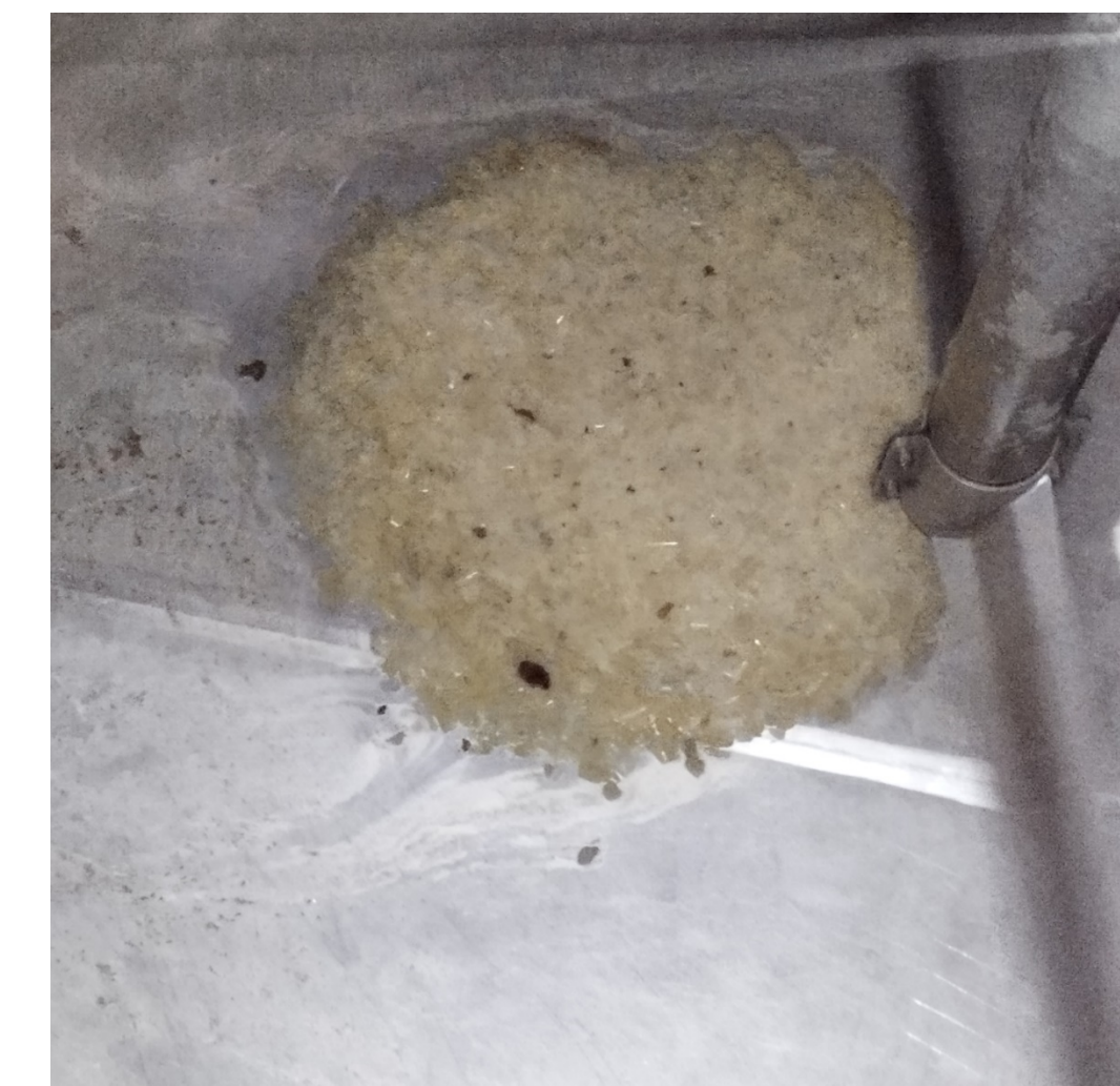
Starch residue from pipes
